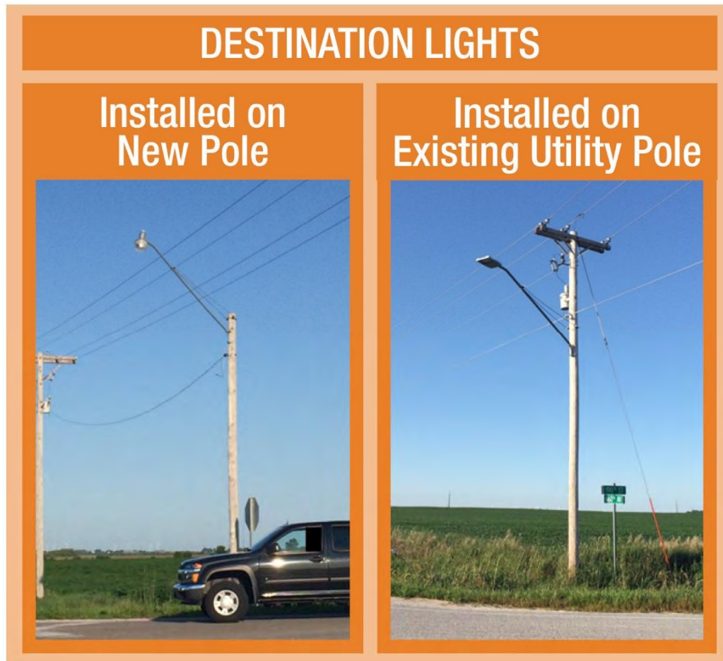
Figure C3 – Destination Lighting Installation Options
